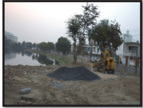
Construction around Urban Pond ( Harni Pond)
